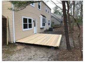
As evidenced in these pictures – an existing Concrete Patio was covered with Pressure Treated lumber – Floating – NON Permanent. Dimensions are roughly  $\sim 12 \times 14$ .
